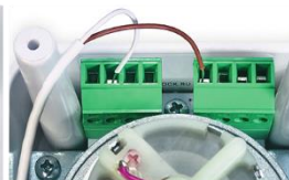
Photo 15. Connecting the sensor to the electric actuator
